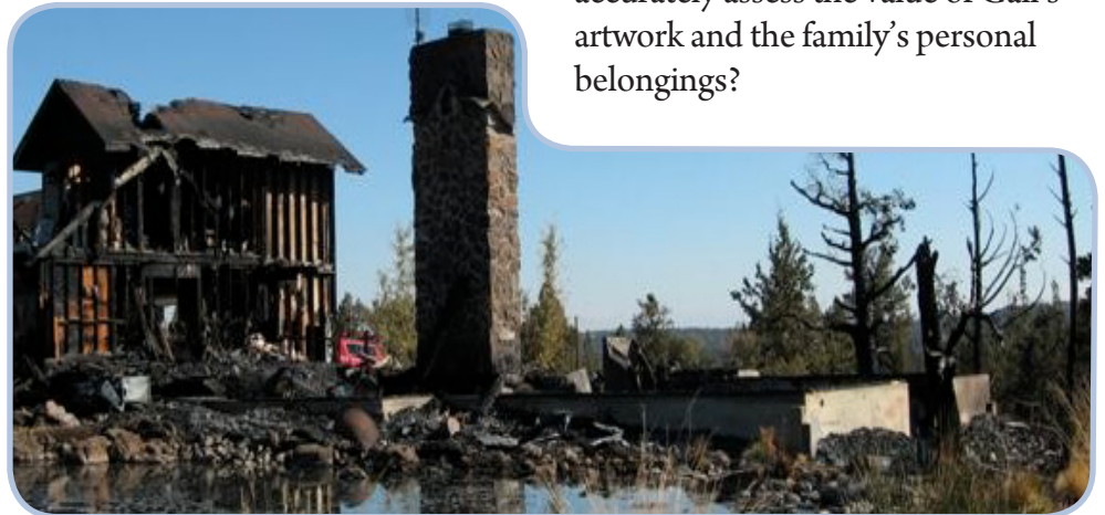
The Davis' home after the fire.
