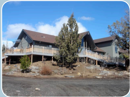
The Davis' home before the fire.
