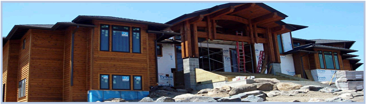
The Davis' home under renovation.
